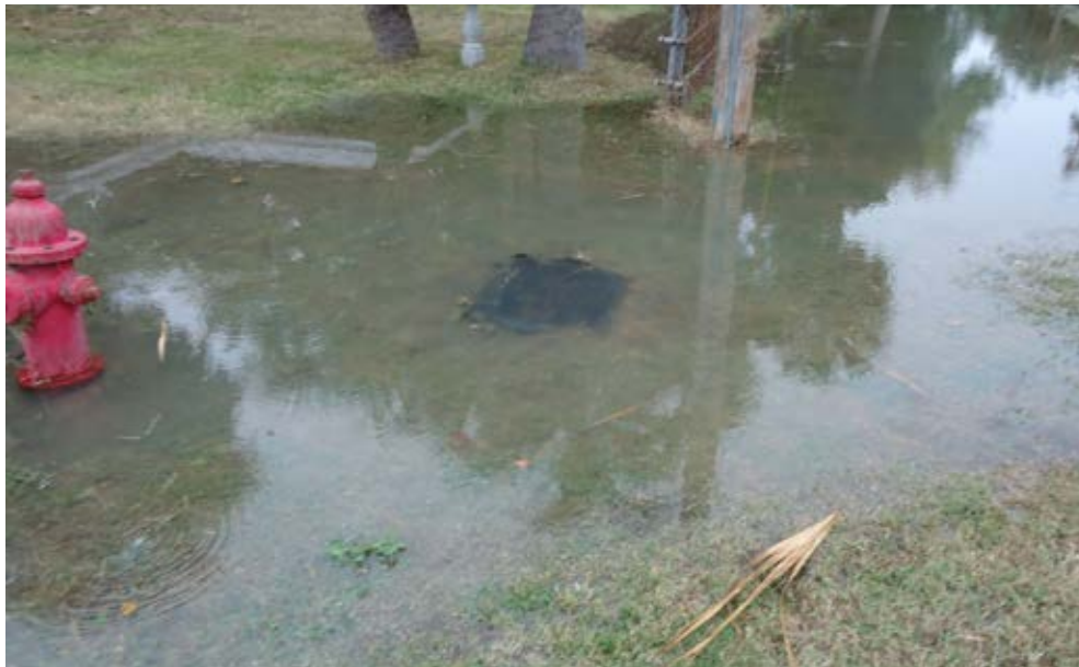
FIGURE 4.6: STORMWATER DRAIN WITH SALTWATER DISCHARGE DURING KING TIDE, NOVEMBER 14, 2012
