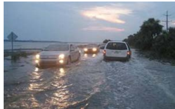
FLOODING ON US 80
