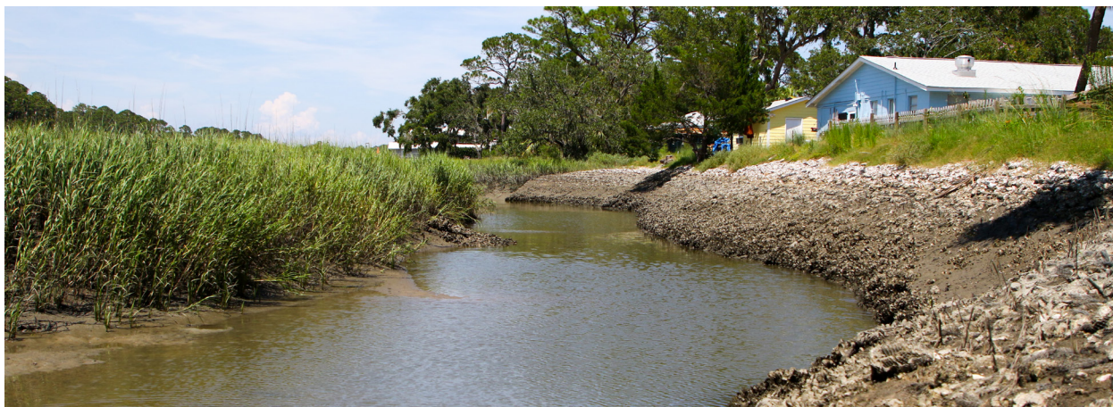
Figure 5.4. The UGA Burton 4-H Center on Tybee Island is stabilizing the shoreline and providing habitat.
