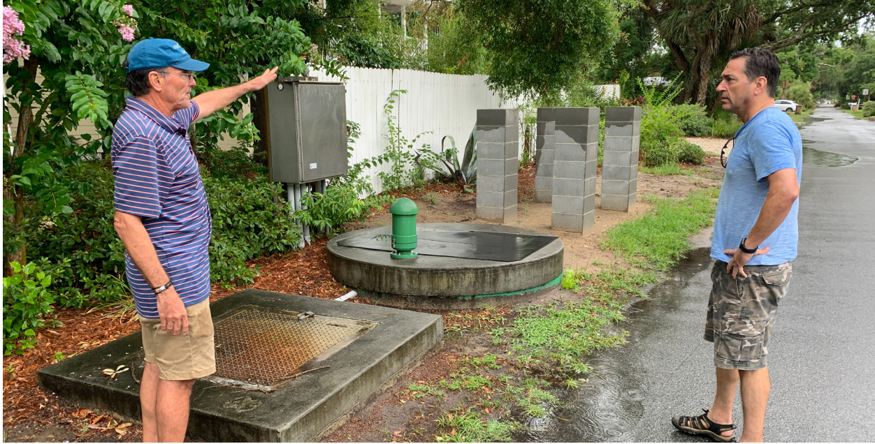
Figure 1. Project members Alan Robertson and Alfie Vick inspect drainage near critical infrastructure.
